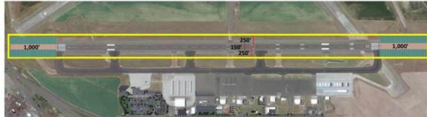
WALLA WALLA REGIONAL AIRPORT (ALW) Runway 2-20 Runway Safety Area
